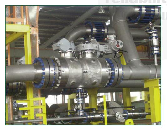
Looking at a traditional hook up, two traditional single 3 piece isolate ball valves and spool piece means a potential of, <u>8 additional leak points</u> (2 from trunnion, 4 from 3 piece design, 2 from spool joints.) Compared to one piece Twinsafe with slipper plate trunnion design.
