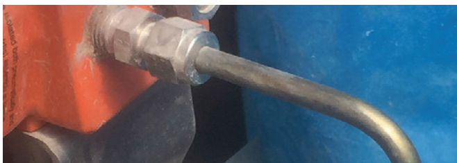
Tungum installed with twin ferrule stainless steel compression fittings, more than 12 years in service with no corrosion issues.
